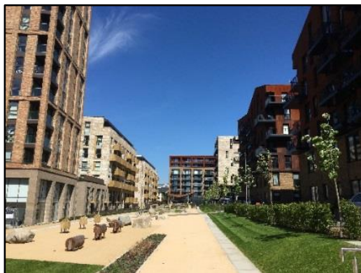
Photo 2.1 (left): Completed housing and Surrey canal Linear Park at Greenland Place, on Plough Way
